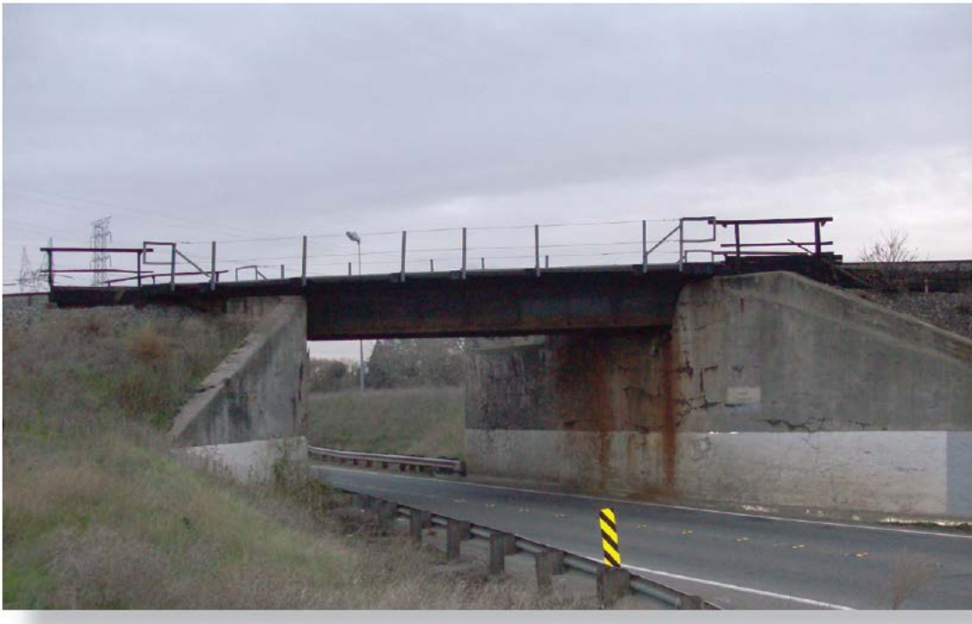
Exhibit 1. Existing Andora Bridge Underpass at Washington Boulevard
